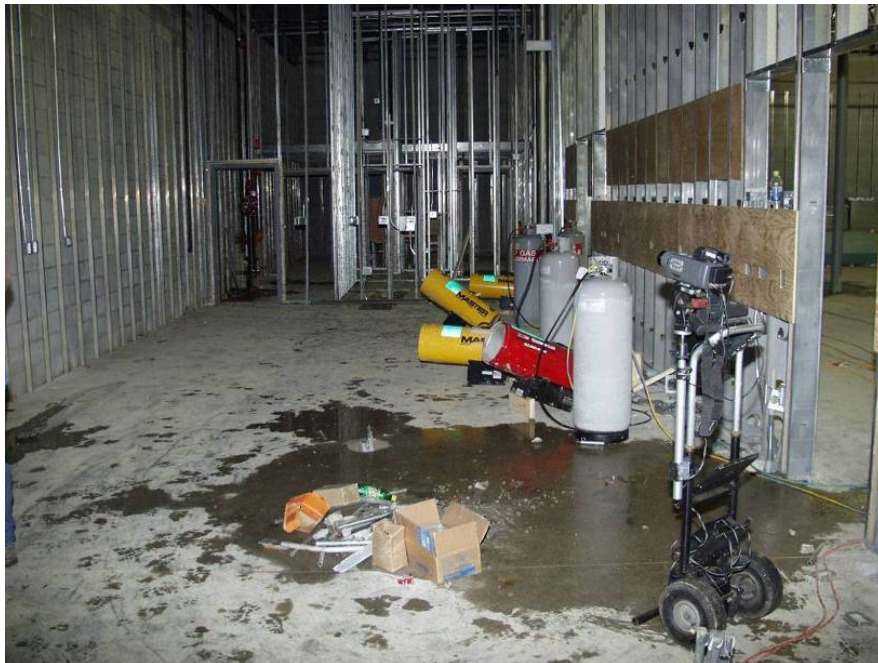
Figure 17. Visual image of a CMU wall being heated.
