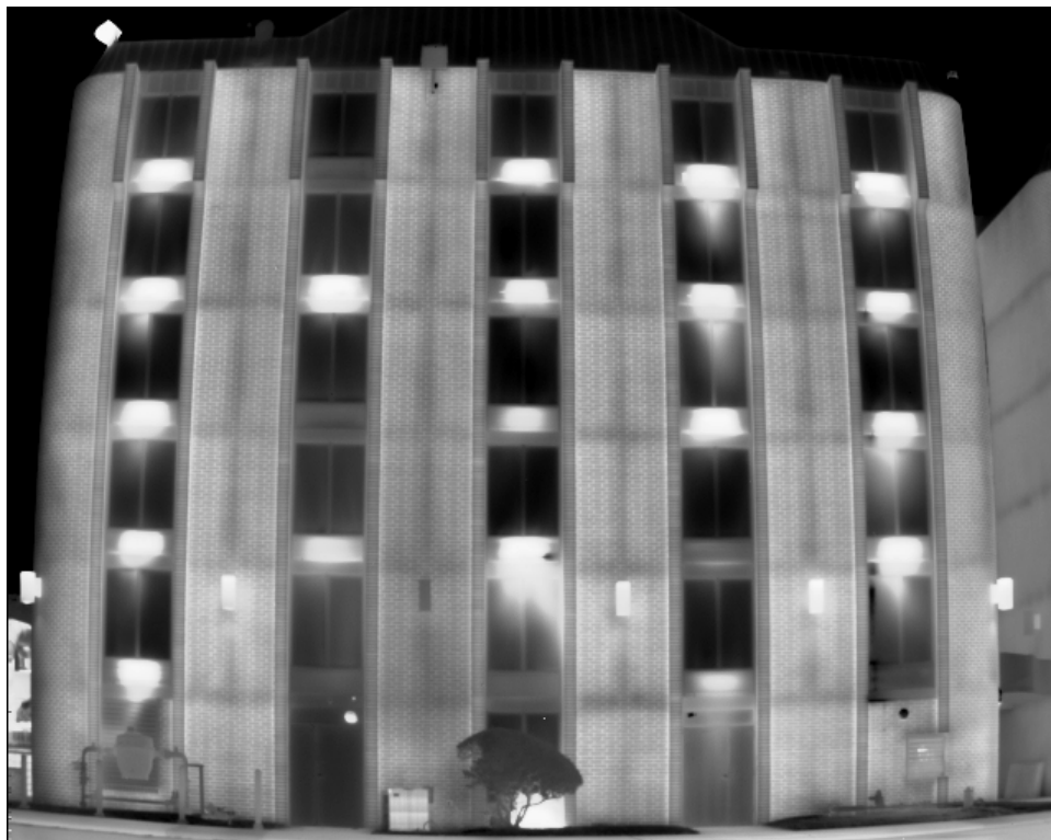
Figure 14. Structural components such as concrete framing can also be seen.
