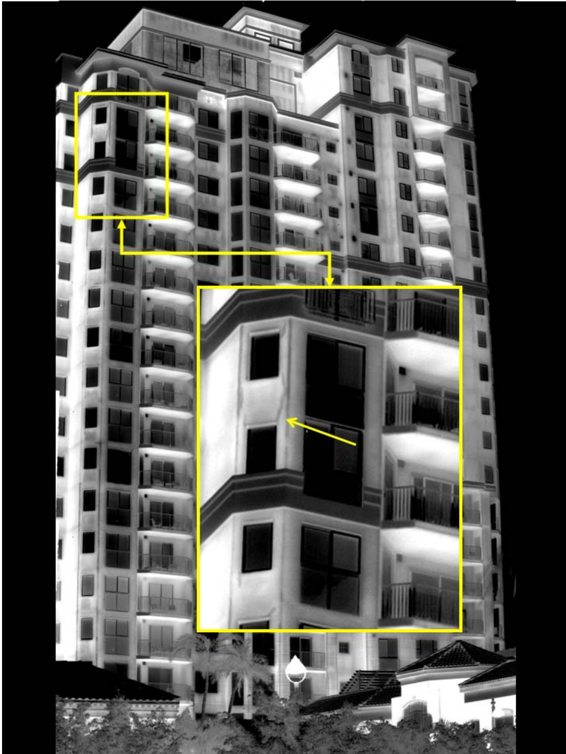
Figure 12. Infrared images of a new condominium with stucco delamination shown.
